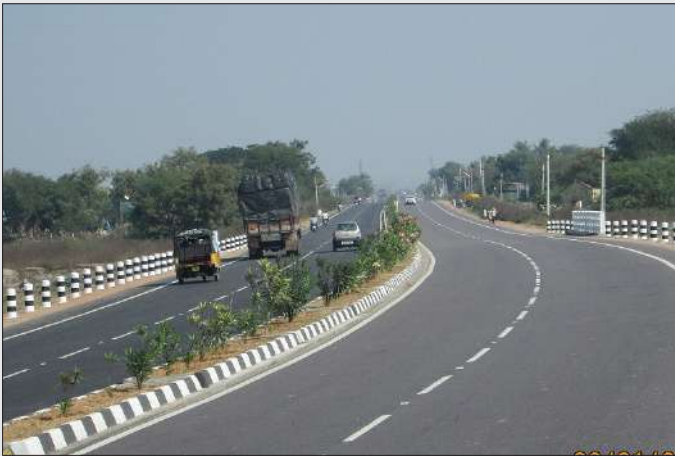
▶ HKR Roadways Limited
